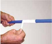
3. When the joint is complete and cool, replace the plastic coat and wrap the joint to give continuity of protection
