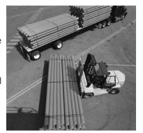
Larger pipe may be off-loaded from vehicles by rolling them gently down timbers, ensuring that they do not fall onto one another or onto a hard, uneven surface.
