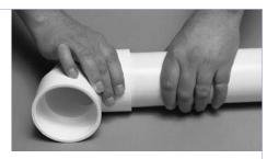
out of round, a satisfactory joint can be made if there is a "net" fit, that is, the pipe bottoms in the fitting socket with no interference, without slop.
